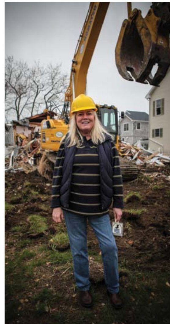
CONSTRUCTION PHOTOS: COURTESY OF KEVIN O’CONNOR
